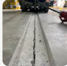
REPAIR OF EXPANSION JOINTS
