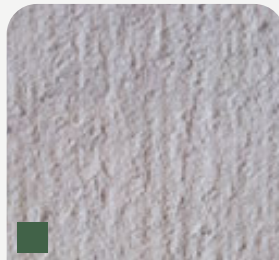
CSP-4 LIGHT SHOT BLASTING
