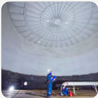
STORAGE TANK BOTTOM PLATES AND ROOF PLATES
