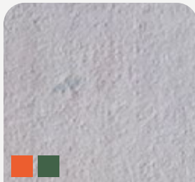
CSP-3 VERY LIGHT SHOT BLASTING OR VERY ROUGH GRINDING
