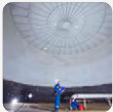
STORAGE TANK BOTTOM PLATES AND ROOF PLATES
