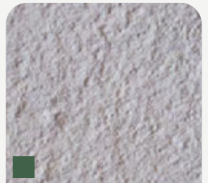
CSP-5 MEDIUM SHOT BLASTING
