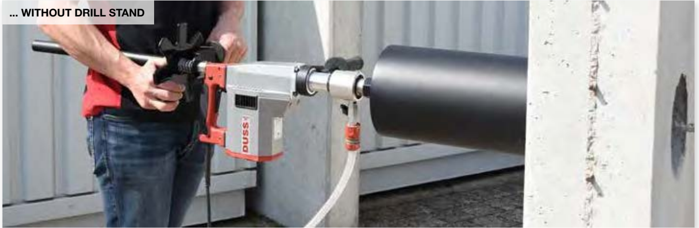
... IN CONFINED SPACES
